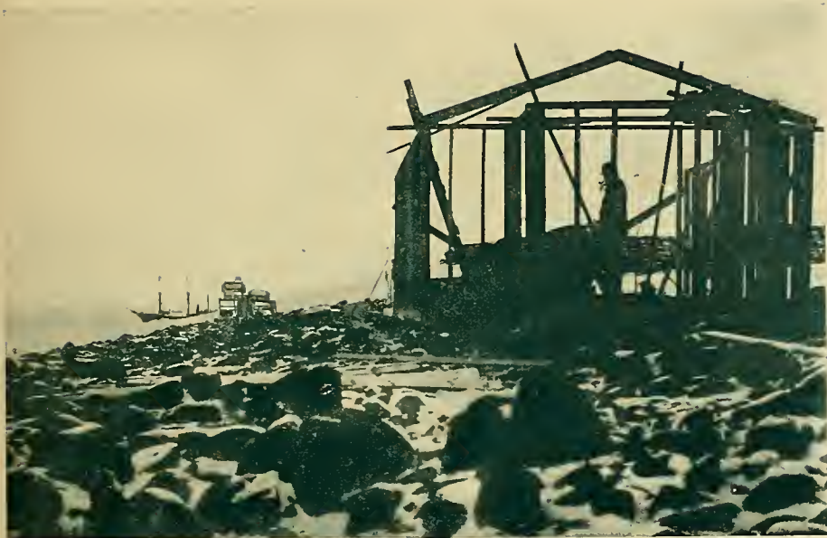
BUILDING A HOUSE AT CAMP ABRUZZI
